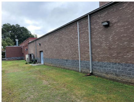
3). North Elevation - Jan 16, 2020
