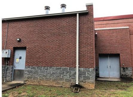
4). North Elevation - Jan 16, 2020
